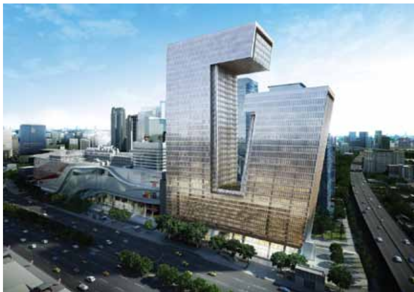
- Photo of G-Land Tower Grand Rama 9 Office Building Project -
